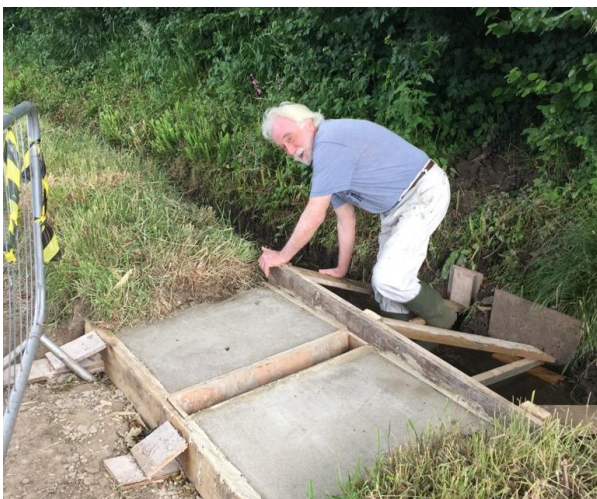
Eddie at work...laying a concrete drain to help with our lane flooding
